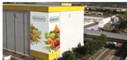
Orogel Production Plant - Cesena, Italy
