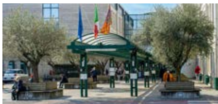
Hospital Fracastoro - S. Bonifacio, Italy
